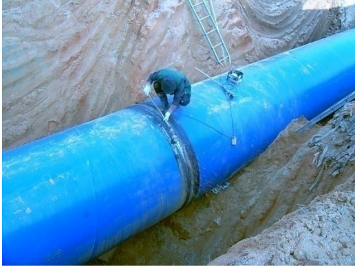
Water steel pipe repair
