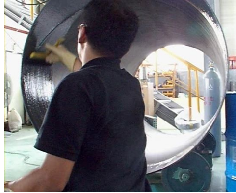
Steel repair coating
