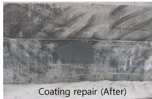
Coating repair (After)
